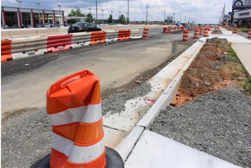
New contractor Lane Construction continues work on curb, gutter and sidewalk work along U.S. 74 East.
